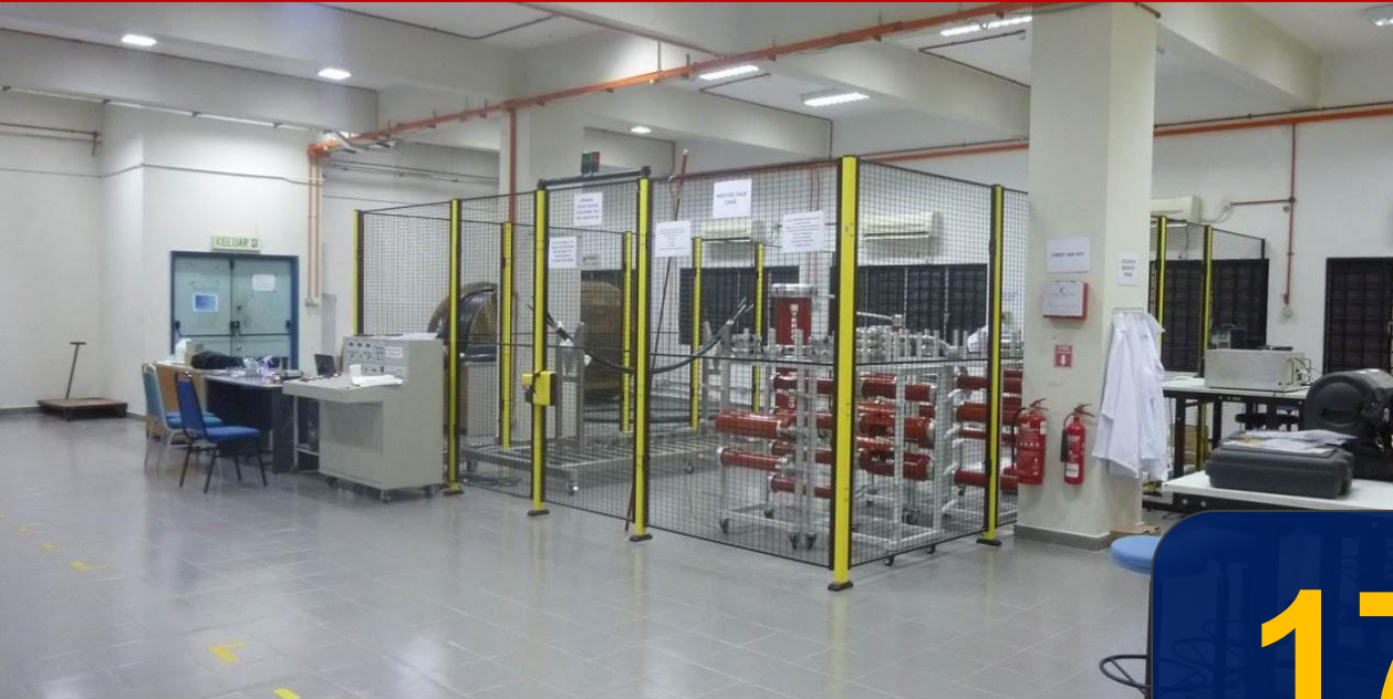
High Voltage Lab
